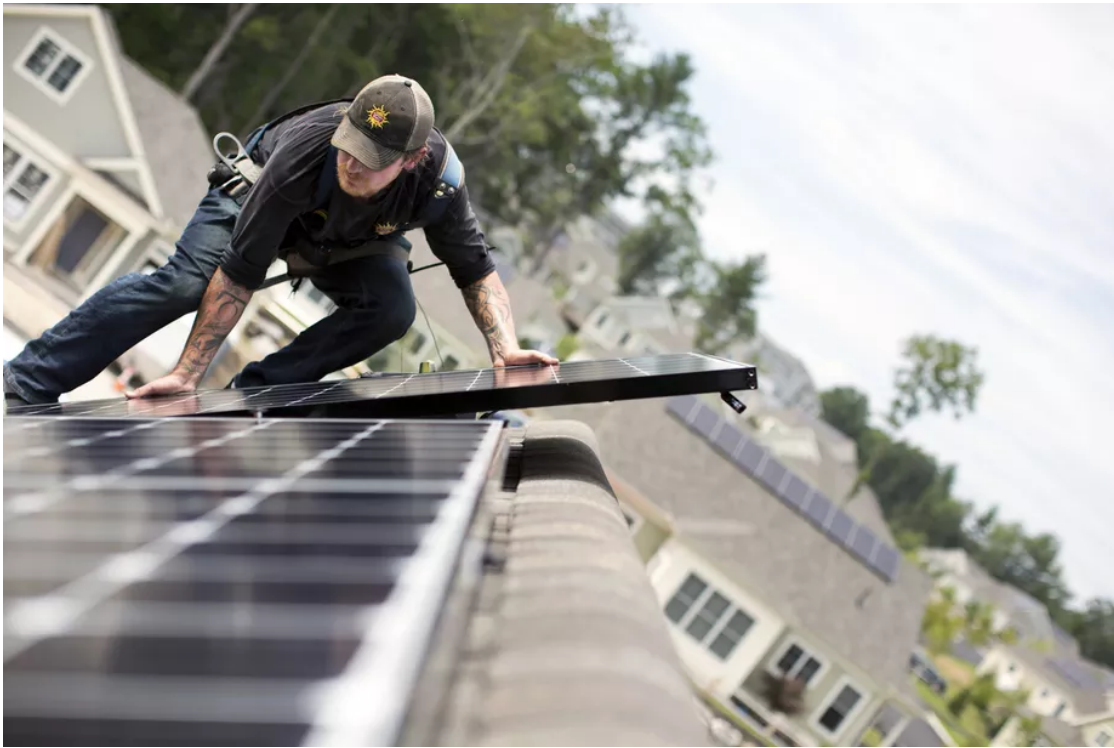
A roofer installs a solar panel on a home in Falmouth, Maine. | Ben McCanna/Portland Portland Press Herald via Getty Images
