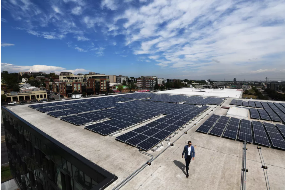
The roof of the 96,000-square-foot “Circa” building on Platte Street in the Lower Highland neighborhood in Denver, Colorado, is covered by solar panels. | Hyoung Chang/The Denver Post via Getty Images
