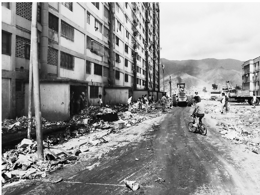
Figure 2. December 23, 1981. Onlookers stand by as bulldozers work on Christmas Eve, removing tons of accumulated trash behind block 6, 23 de Enero. Giorgio Lombardi/ El Nacional .
