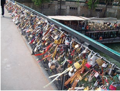
Figure 1.2. Padlocks on the Pont Echevren behind Notre Dame Cathedral, Paris
